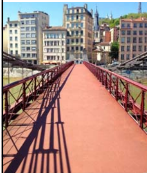
1 Passerelle Saint Vincent
